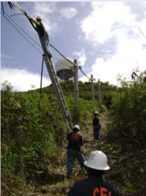
Tower & Aerial Installation
